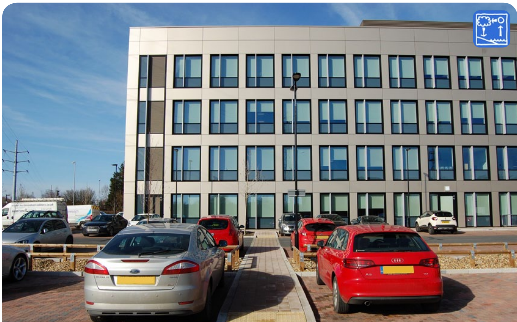
Maurice Wilkes Building, Cambridge Car parking bays with permeable paving which discharge surface water run off into the adjacent planted swale feature.
