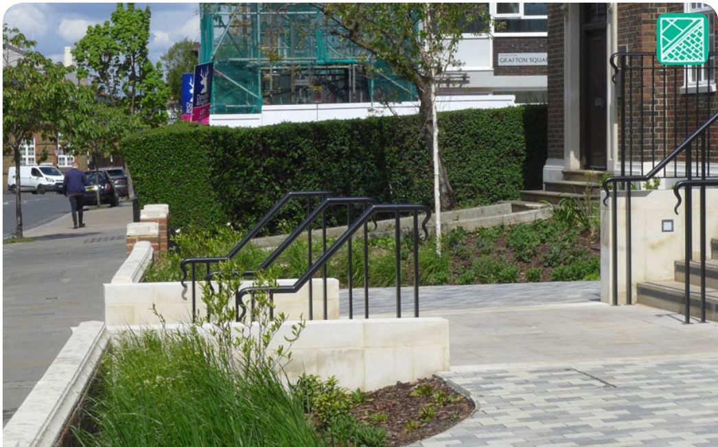
Maritime House, Clapham A functional Part M compliant pedestrian entrance to this multi occupancy office building.
